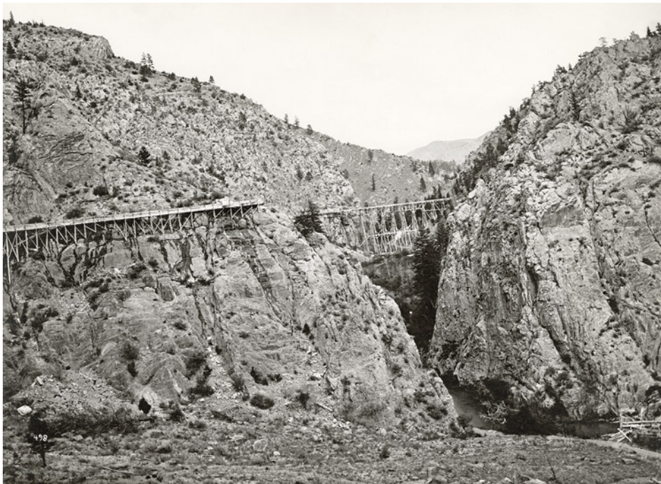
Figure 8. The flume taking water from Trout Creek to the sapphire and gold mining operations at the Missouri River. In this view, the flume is crossing Trout Creek itself, with the water taken from further upstream. Photo by W.H. Jackson during the 1869–1871 Hayden Survey. Lot 032 B5F09.03a Trout Creek Flume, Montana Historical Society Photograph Archives.
