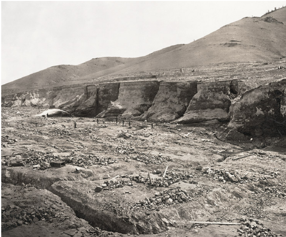
Figure 9. Hydraulic mining at French Bar along the Missouri River between 1870 and 1879. PAC 97-32.9, Montana, Montana Historical Society Photograph Archives.
