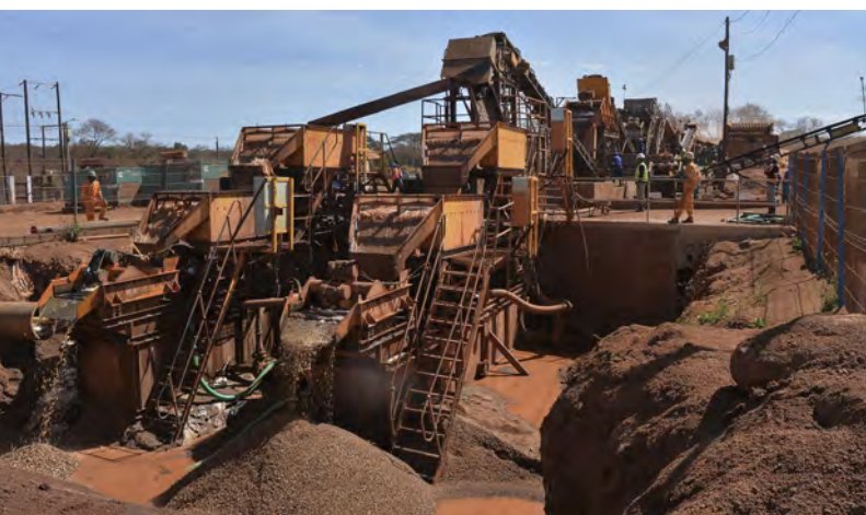
Figure 5. Jigs at the MRM washing plant. The washing capacity of this installation is reportedly 130 tons per hour. Photo by Vincent Pardieu/GIA.
